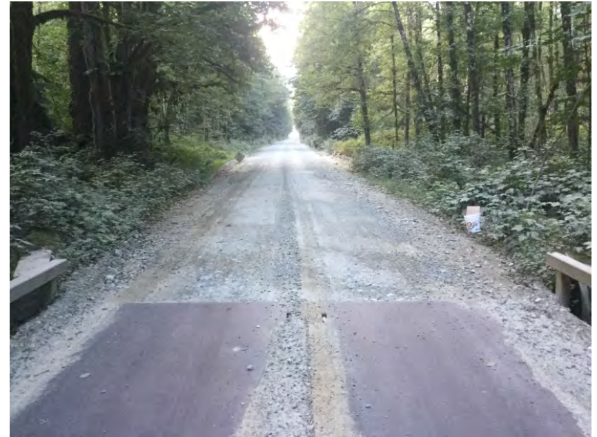
Left Approach Facing Away From Bridge
