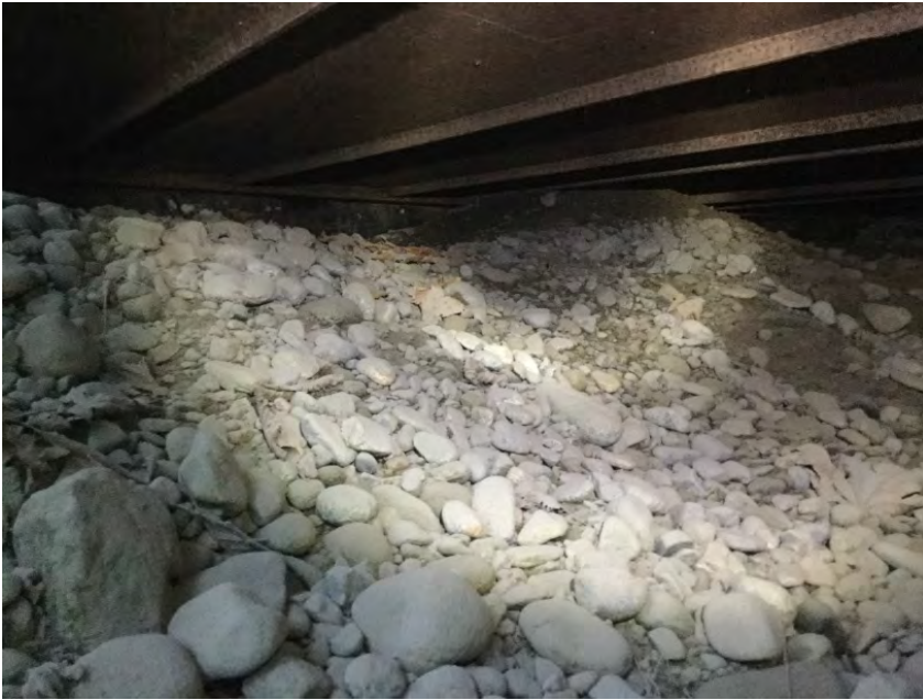
Left Bank Abutment
