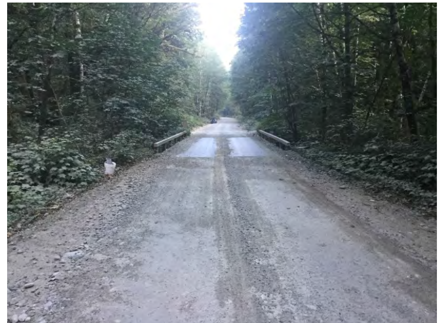
Left Approach Facing Bridge
