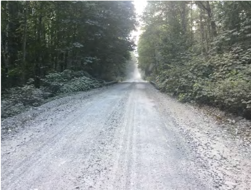
Right Approach Facing Bridge
