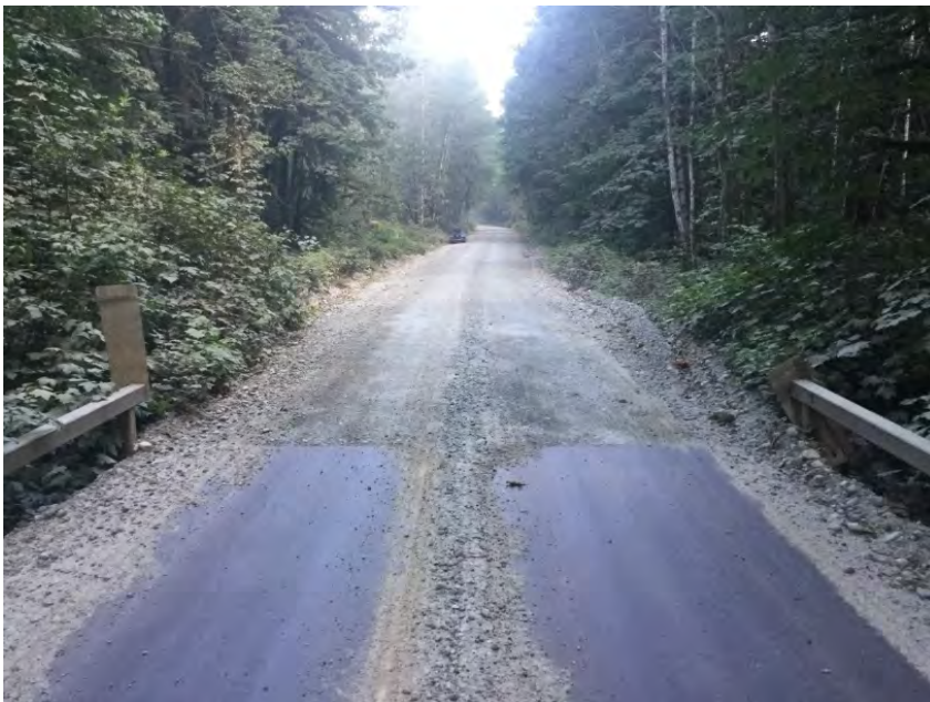
Right Approach Facing Away From Bridge
