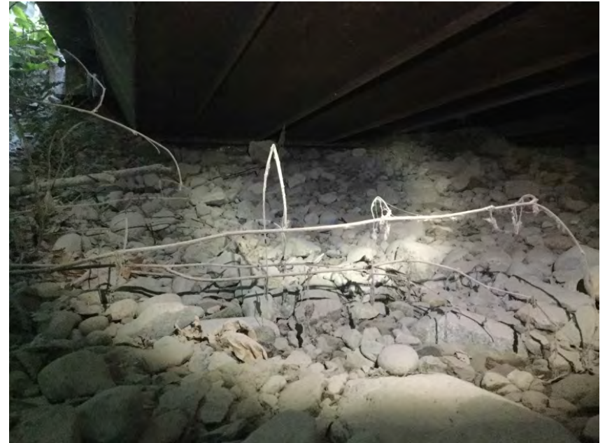
Right Bank Abutment
